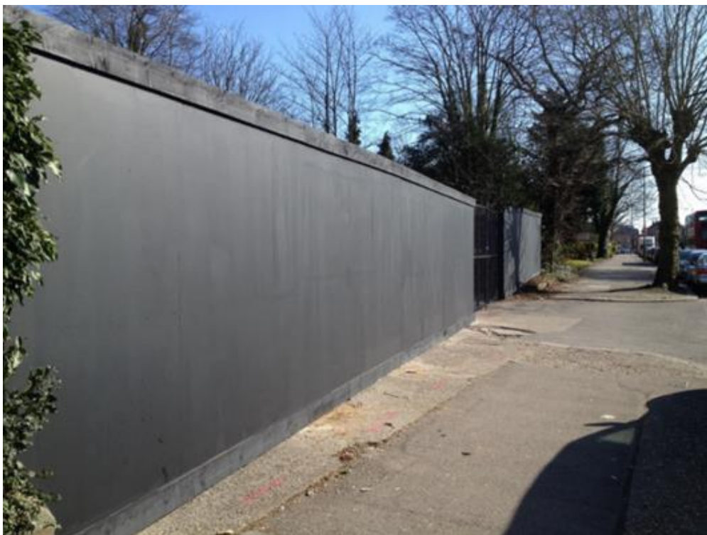
Image 6: Example of suitable hoarding
